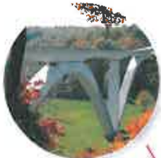
NATCHEZ TRACE PARKWAY BRIDGE
